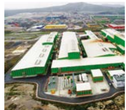
Steel Factory (Turkey)
