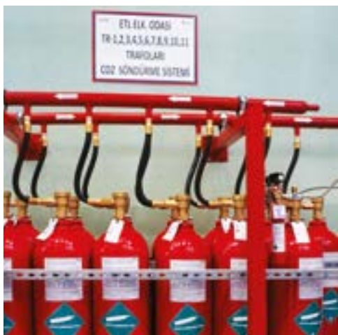
Sample of High Pressure CO 2 System
