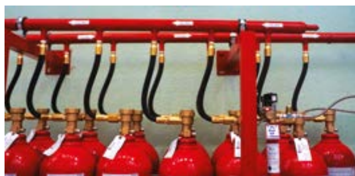
Sample of 200 Bar Inert System
