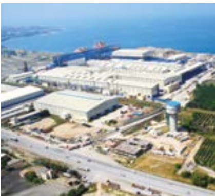
Steel Factory (Turkey)
